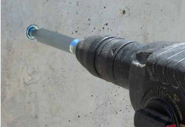
Anchor being set with SDS setting tool.
